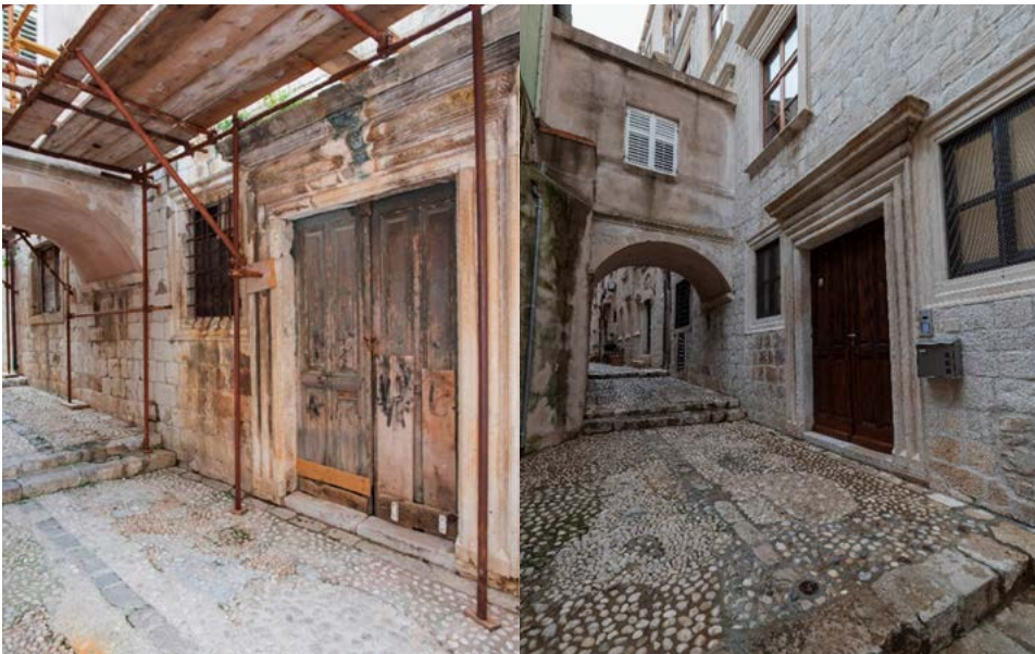
The main entrance and façade before and after reconstruction.
