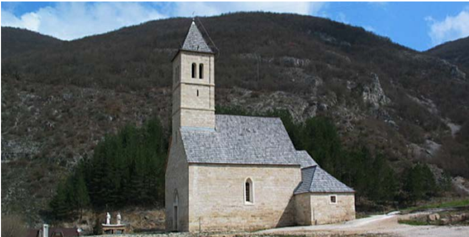
Fig. 20. Catholic Church of St. Ivo in Podmilačje after reconstruction.
