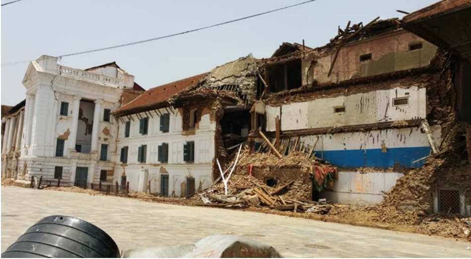
Fig. 5. The Hanuman Dhoka palace museum located in the World Heritage Monument Zone of Kathmandu valley World Heritage Site in Nepal was extensively damaged due to earthquakes in 2015. It was a challenge to rehabilitate both the historic buildings and the museum collections.
