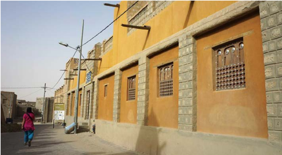
Renovation of the facade of the ESSAYOUTI library using Bourem earth and limestone alhor rekindled interest in local building materials (Photo: Timbuktu Cultural Mission).
