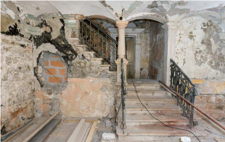
The entrance hall before reconstruction.
