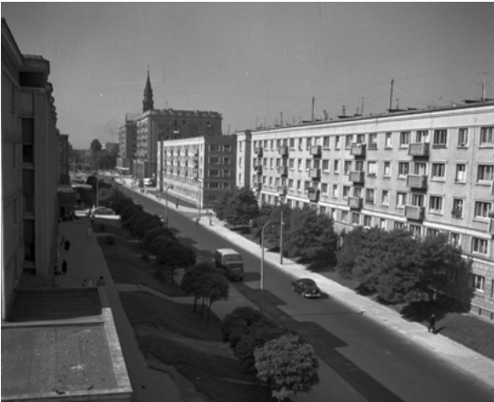
Fig. 6a – 6b. Muranów, Nowolipki Street (5a. 1949, photo by J. Bułhak; 5b 1961, photo by J. Bułhak). Archive of National Heritage Board of Poland.
