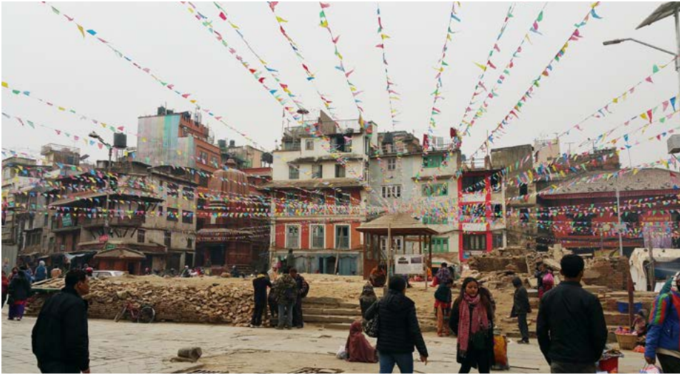
Fig. 6. Kashthmandap; one of the important heritage structures located in one of the World Heritage Monument Zones of Kathmandu Valley World Heritage Site in Nepal collapsed due to 2015 earthquakes causing death of many more people. The engineers and heritage professionals argued long over the right approach for its reconstruction as the former emphasised safety while the latter insisted on protection of heritage values.
