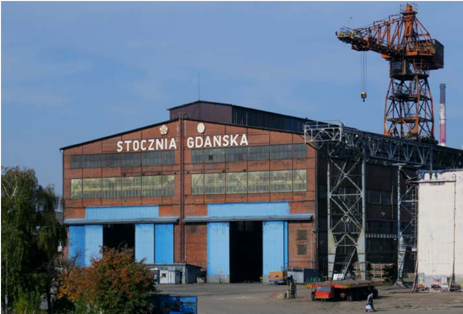
Fig. 9. Gdańsk, Historic Gate No. 2 of the former Gdańsk Shipyard, 2018. Photo by Tomasz Błyskosz, the archive of National Heritage Board of Poland.
