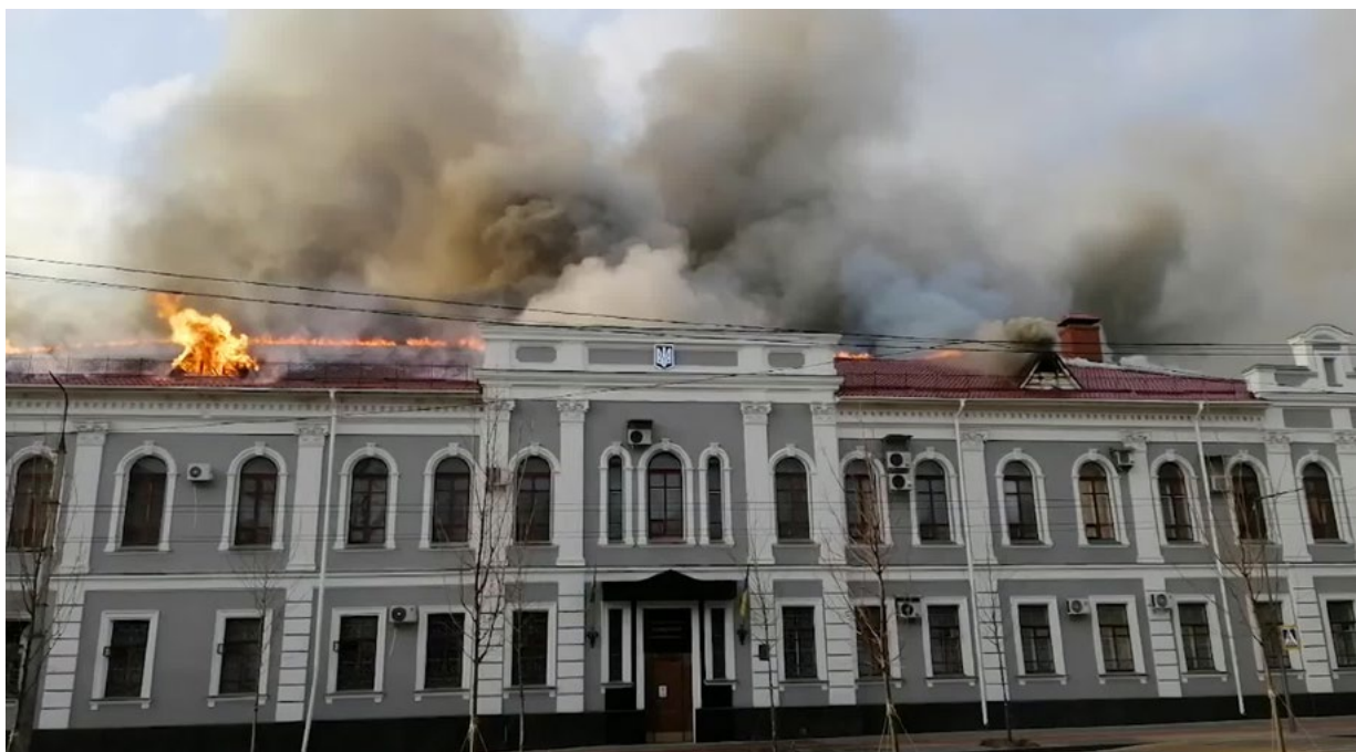
Fire in the building of the Archives Department of the Security Service of Ukraine (SBU) in the Chernihiv region on 25 February 2022.
