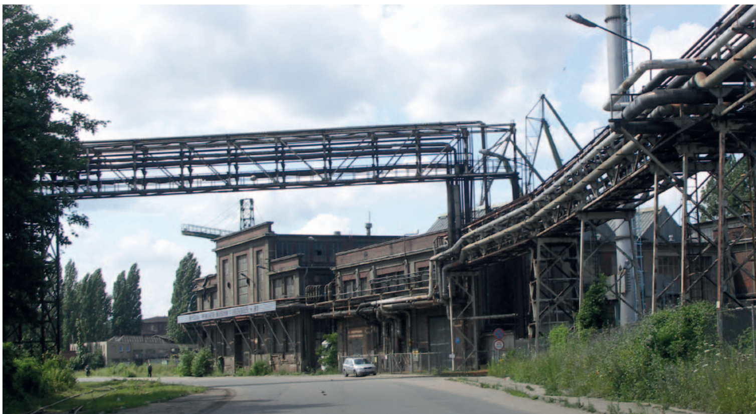
49. The R3 department's machinery and equipment overhaul hall (deep, higher) and boiler room (64B - on the right). In the foreground, on the left, the preserved section of the shipyard railway line, Narzędziowców St. and a now defunct section of the flyover with pipelines for the transmission of, among other things, industrial gases, 2009. Photo: T. Błyskosz, National Institute of Cultural Heritage archives
