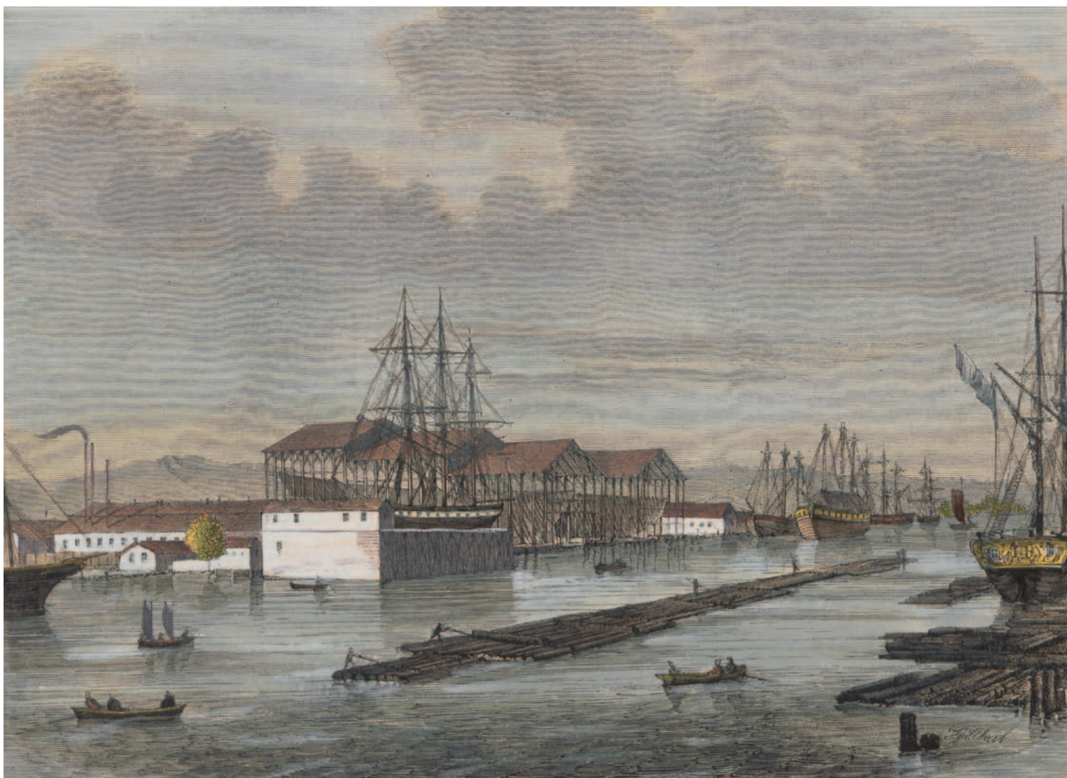
7. Prussian Royal Naval Shipyard in Gdańsk (German: Königliche Werft Danzig) – the first state shipyard of Prussia and Germany – a few years after its foundation. In the centre, the Klawitter floating dock and the covered slipways with the hulls of the ships under construction are visible. In the foreground, wooden logs joined together to form rafts – raw material transported by water to the port of Gdańsk or for the shipyards, 1861. Fig. NN according to a drawing by J. Gottheil, collection of the Polish Academy of Sciences Gdańsk Library.
