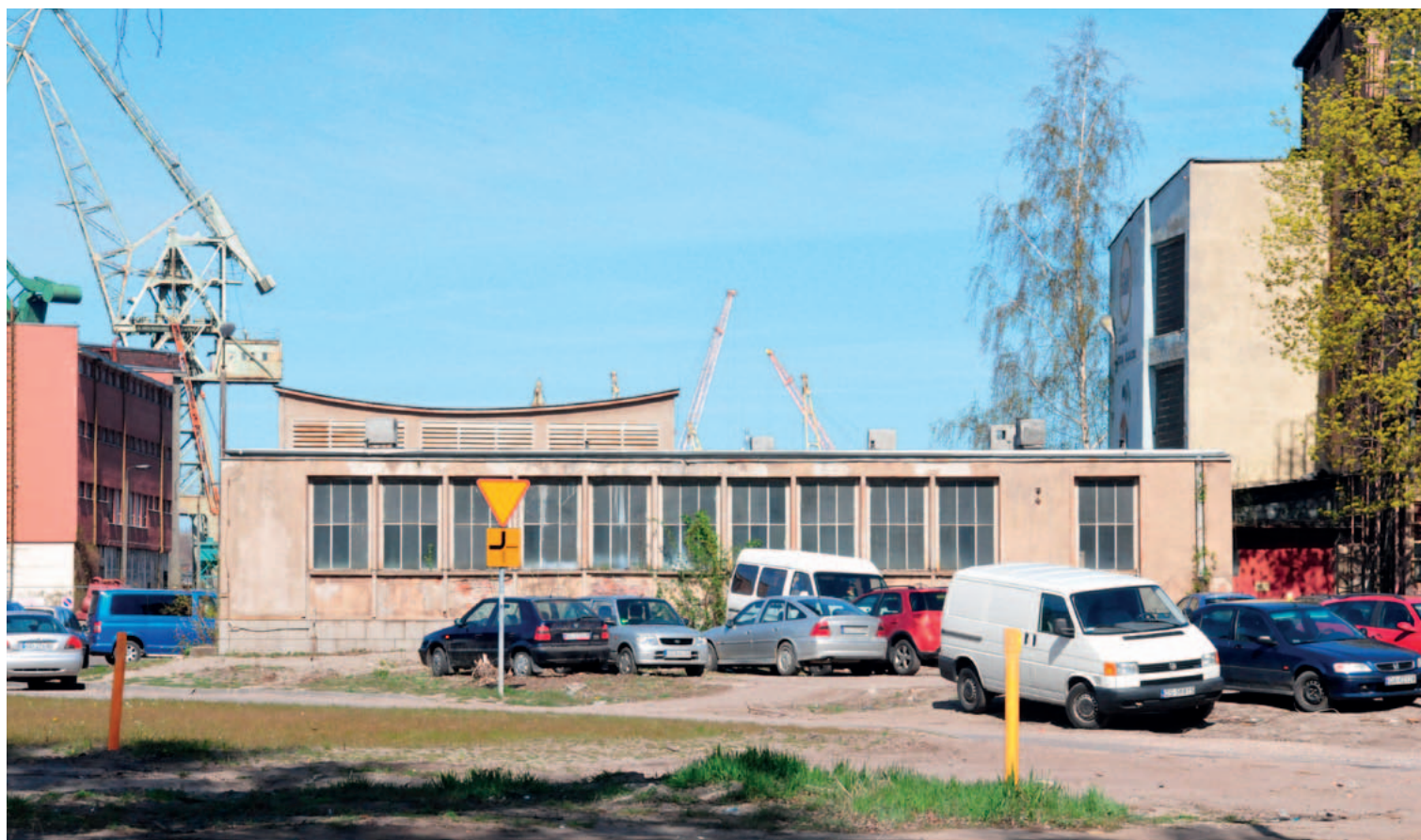
57. A9 transformer and distribution substation – object 347A. On the right, the defunct building of the tube and pipe manufacturing department W2, on the left in the background, the social and office building of the department W4, 2015. Photo: A. Trzeciak, collection of the author
