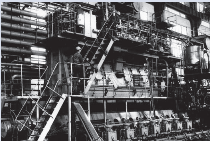
20. The Gdańsk marine engines during construction at the Gdańsk Shipyard. These ships' main propulsion units were built under licence from the Danish company Burmeister & Wein, 1970s. Photo: Z. Mirota, State Archive in Gdańsk collection
