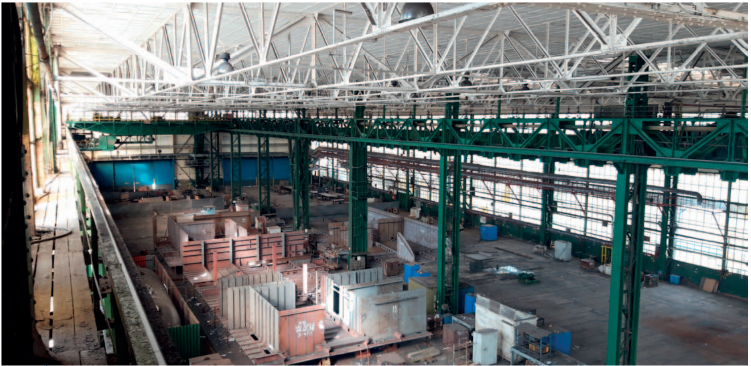
28. Interior of the hull section prefabrication hall (3B) of the Gdańsk Shipyard – the so-called hull workshop. Here, machined plates and angles were assembled into sections – parts of the ship’s hull. Visible prefabricated elements of ship sections, 2020. Photo: T. Błyskosz, National Institute of Cultural Heritage archives
