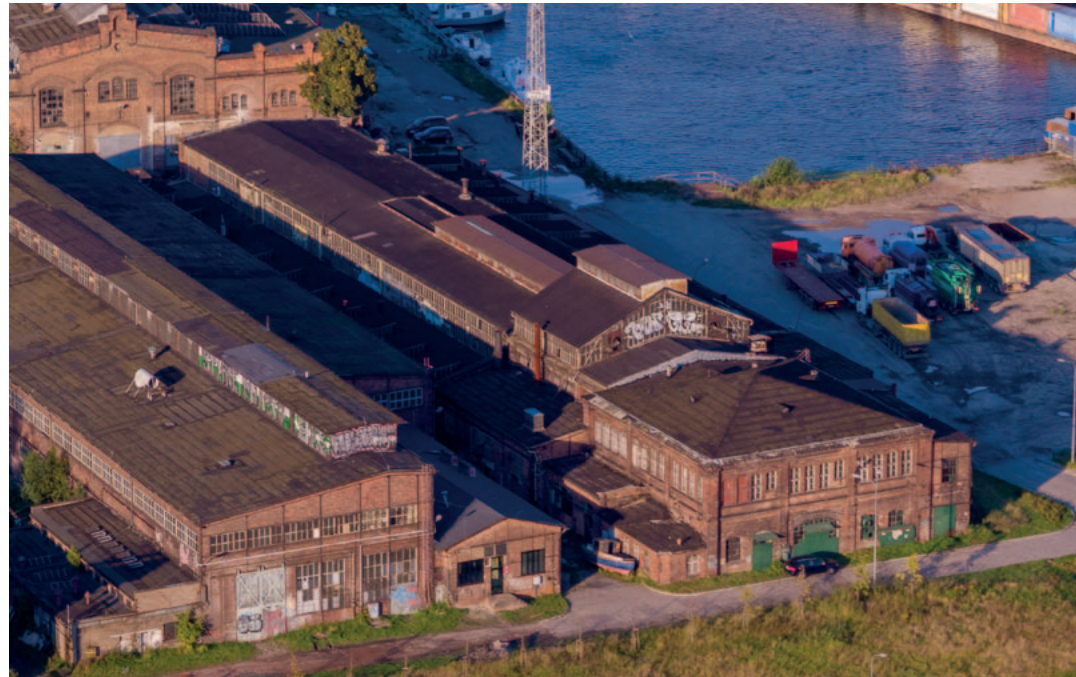
73. The forge hall of the Gdańsk Shipyard (36A) together with the office area (36Aa; right). Building 36A maintained its function as a shipbuilding forge workshop from its construction in the 1880s until 2016, 2018. Photo: M. Czacharowski, National Institute of Cultural Heritage archives
