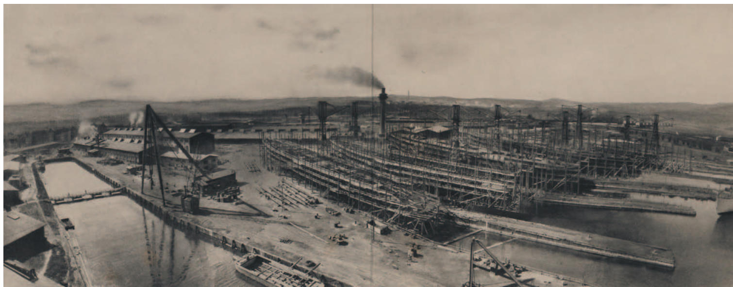
8. Ferdinand Schichau Shipyard in Gdańsk. In the centre, ramps; on the left, a pool used to fit out vessels. Behind it, industrial buildings, partly preserved today, ca. 1912. Photo: NN, public domain
