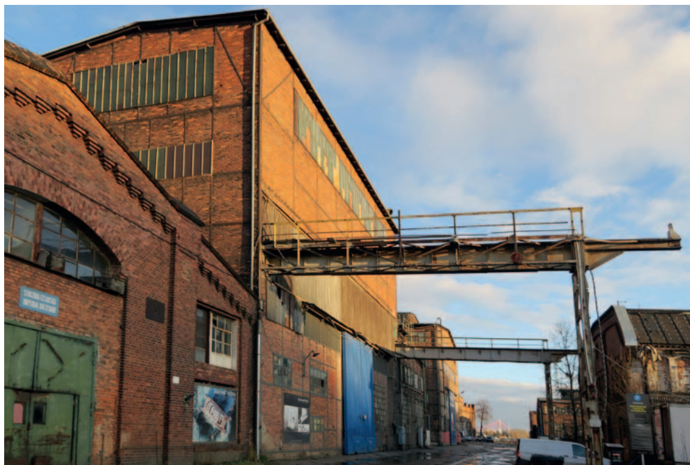
66. South massing of the boiler house (34A) including the external flyover of the crane for material and product handling, 2018. Photo: T. Błyskosz, National Institute of Cultural Heritage archives
