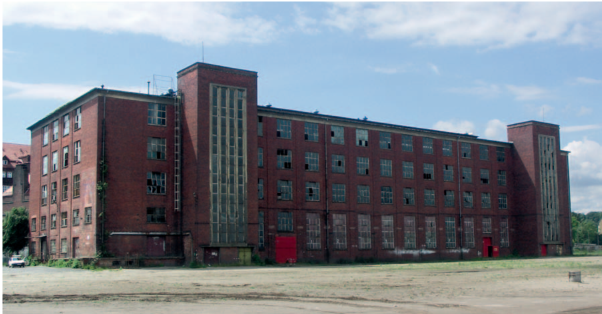
80. Site A main warehouse building (89A). Next to it was a sheet metal warehouse. The halls of the K2 Hull Assembly Department were previously in the empty area in the foreground, 2009. Photo: T. Błyskosz, National Institute of Cultural Heritage archives
