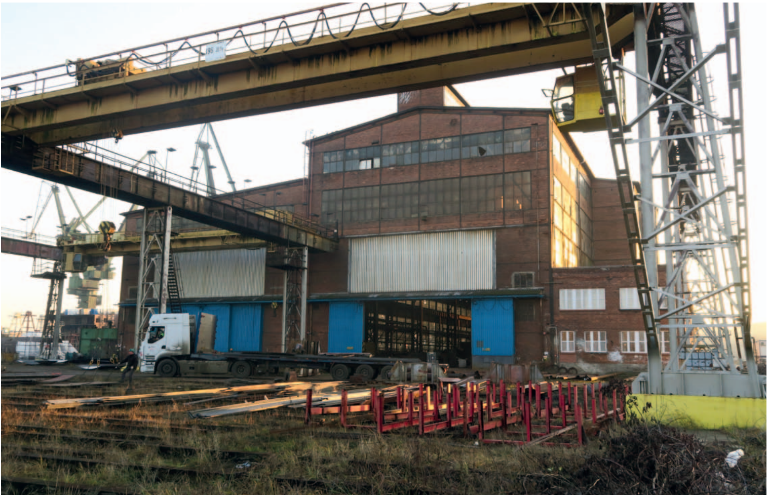
39. In the foreground, the hull materials picking yard with crane flyovers and cranes. In depth, north elevation of the hull section prefabrication hall (3B), 2019. Photo: T. Błyskosz, National Institute of Cultural Heritage archives
