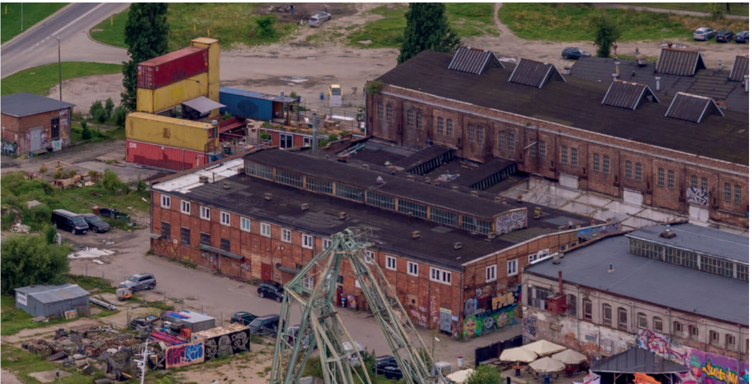
46. Hall with wood drying room (31B) of the Carpentry Department W5 of the Gdańsk Shipyard, 2018. Photo: M. Czacharowski, National Institute of Cultural Heritage archives
