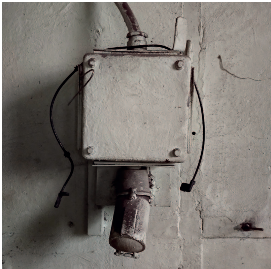
44. Located in the electric carriage hall is the distinctive, massive socket for charging the batteries of the yard's electric carriages, one of the few surviving, 2022. Photo: A. Trzeciak, collection of the author
