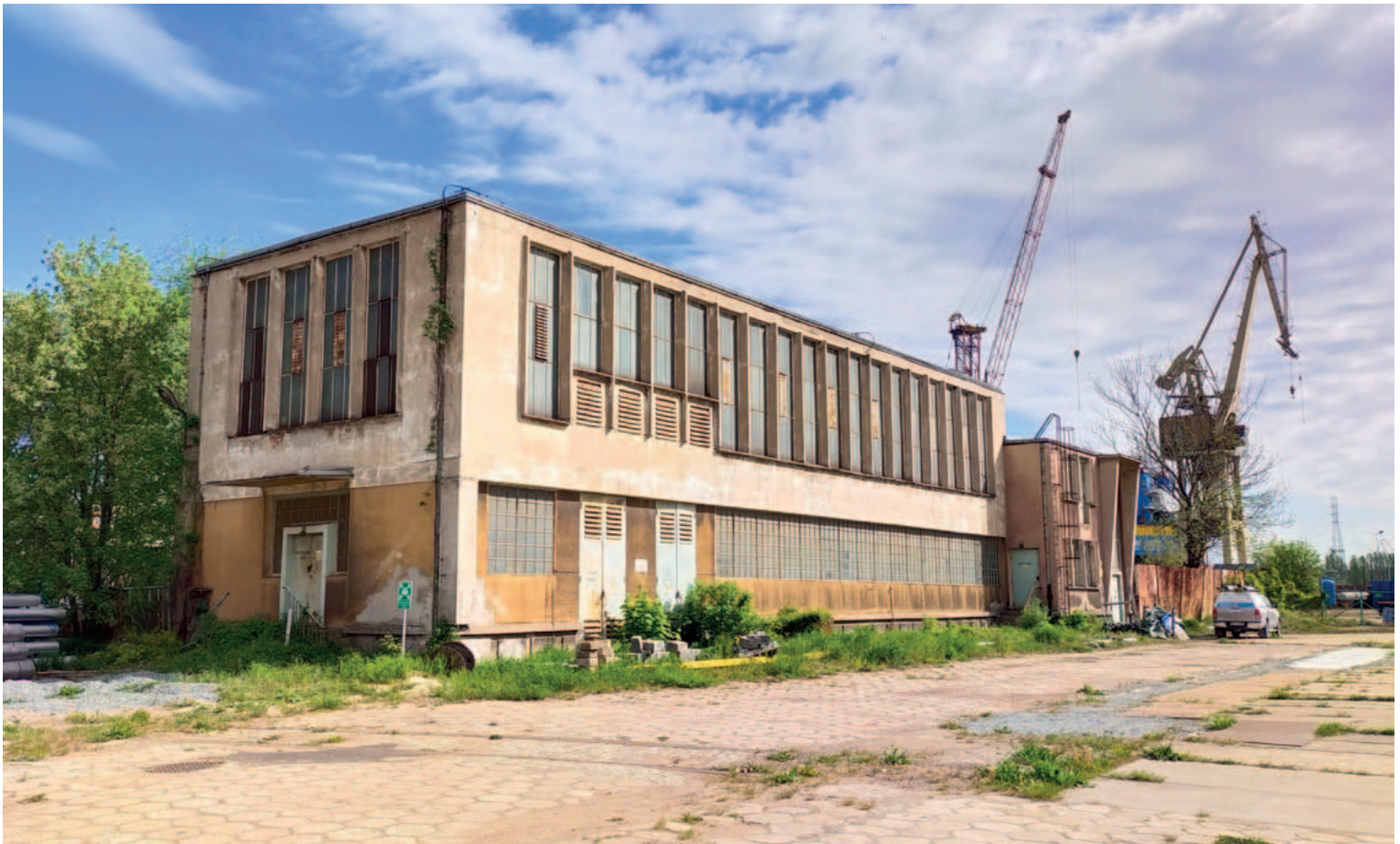
36. Building of the main electrical switching station at the Gdańsk Shipyard. An example of Polish post-war architecture with an industrial character, 2022. Photo: A. Trzeciak, collection of the author
