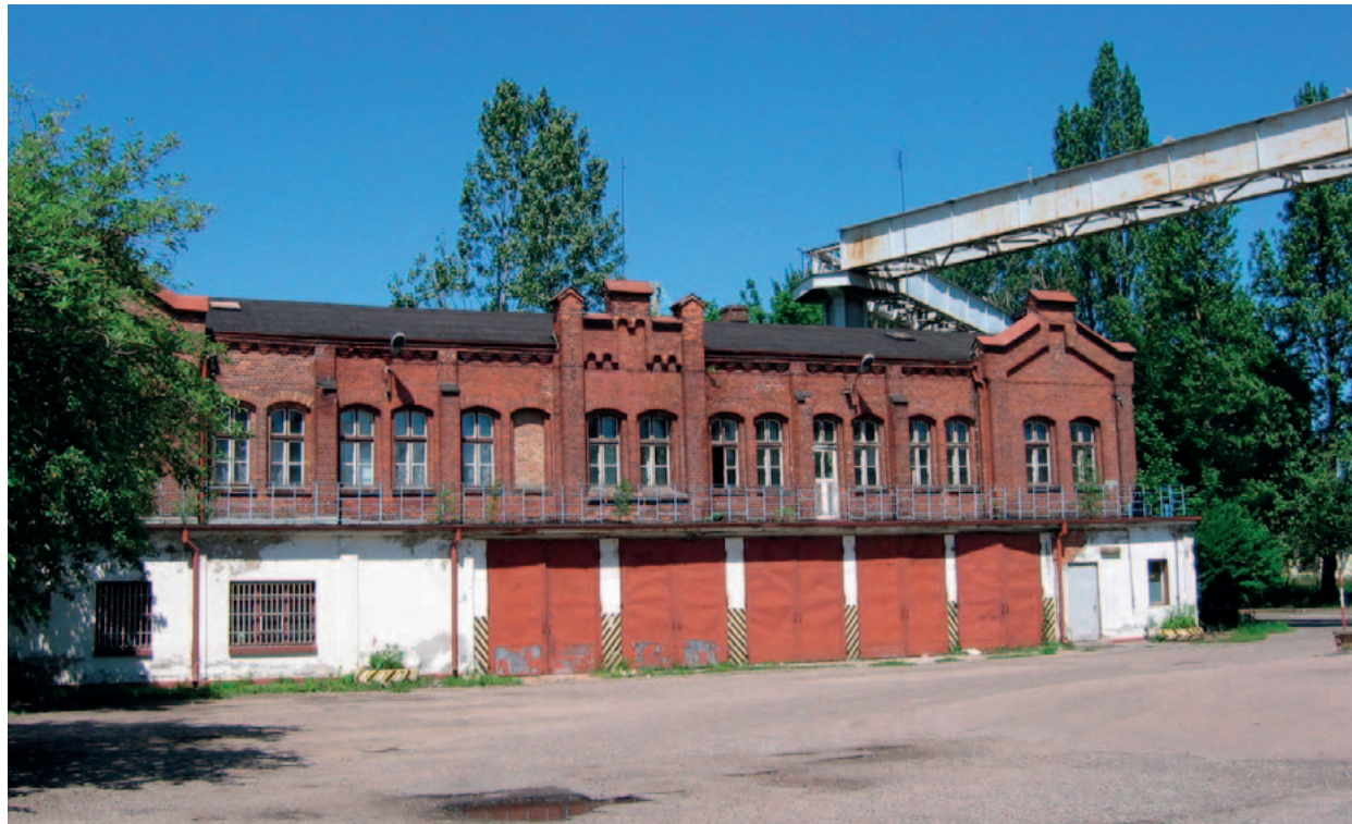
83. Company Fire Brigade building – fire station. The building has served this function since its inception in the 2nd half of the 19th century, 2018. Photo: T. Błyskosz, National Institute of Cultural Heritage archives
