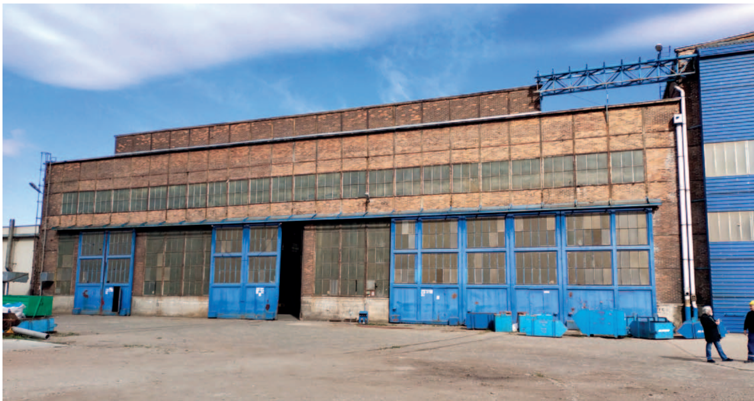
38. Part of the eastern elevation of the sheet metal machining hall (4B). Visible gates closing the three working passages, 2022. Photo: A. Trzeciak, collection of the author
