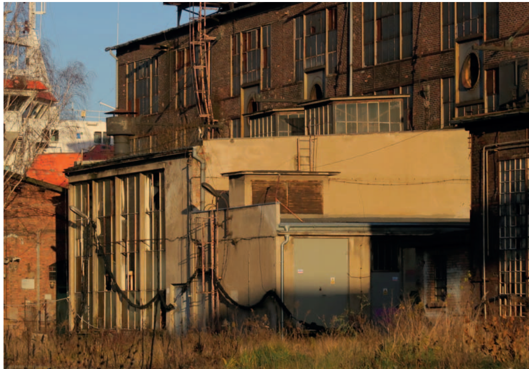
63. Attached to the brick engine assembly hall (28A) is a rendered engine and fuel station building. In the lower part (with a characteristic vent on the roof) there is a transformer substation (A10), 2018. Photo: T. Błyskosz, National Institute of Cultural Heritage archives
