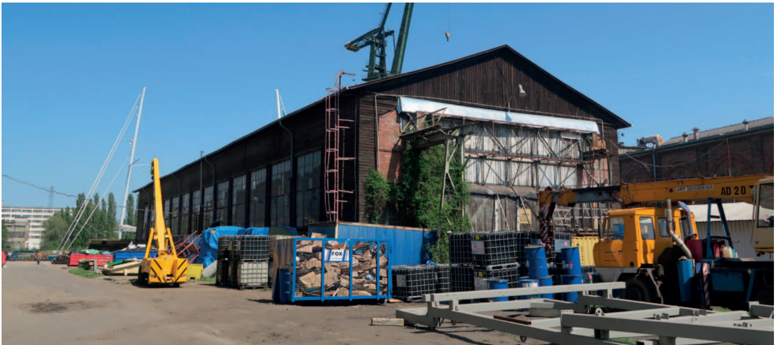
69. Locksmith hall 1 (41A). The wooden cladding of the masonry, not used in other shipyard buildings, draws attention, 2018. Photo: T. Błyskosz, National Institute of Cultural Heritage archives
