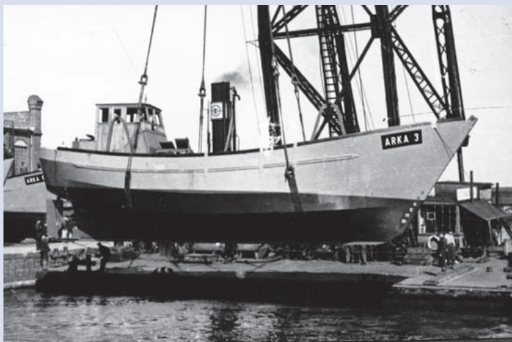
10. Ark 3 – type K 17 steel cutter (39 DWT), 1949. The world's first all-steel fishing boat. Polish shipyards built nearly 200 similar vessels following to this design, ca. 1949. Photo: NN, State Archive in Gdańsk collection
