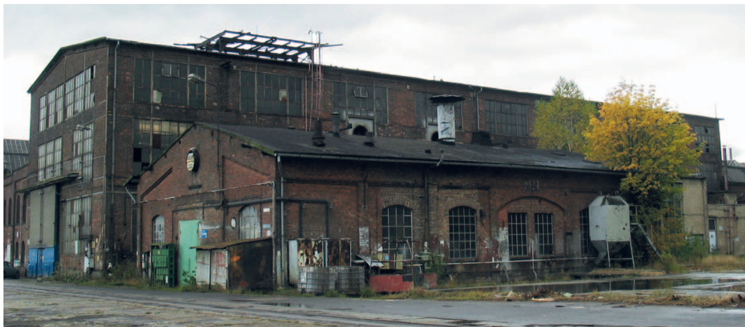
59. North-west elevation of the hardening plant building. Behind it, engine assembly hall 28A, 2005. Photo: T. Błyskosz, National Institute of Cultural Heritage archives
